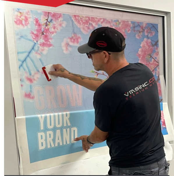
Installing frosted window graphics
